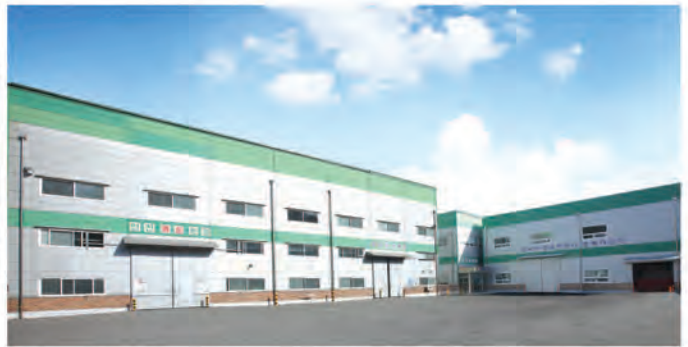
• Eumseong Plant #2 (Daeji Corporation)
